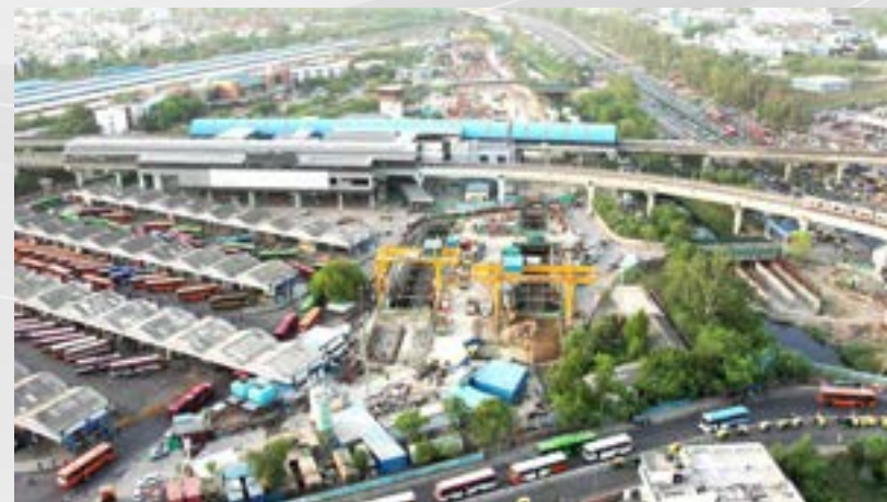
October 2022 – RRTS TBM launching Shaft 01 at Anand Vihar
